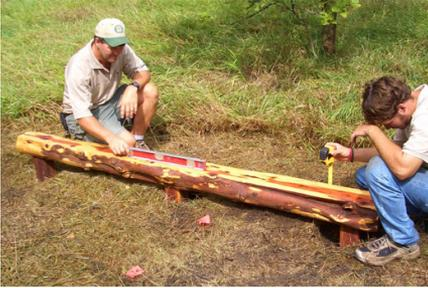
**Note:** According to CPSC safety guidelines, the highest designated play surface should be no more than 12" above the compacted safety surfacing level.
