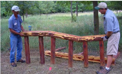
**2** Lower the balance beam into the footing holes. Use scrap wood to brace into position if necessary.
