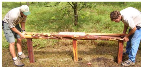
**3** Make sure that the highest designated play surface is the proper height. Also check to see that the beam is level and plumb in footings. You may need to fill the holes with additional material as needed to fit post.
