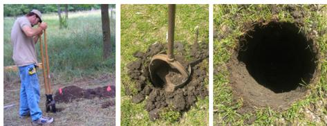
**8** Using the tamping post, compact the soil at the bottom of the footing hole.
