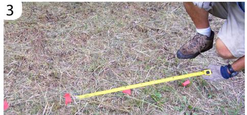
Each log step is approximately 12" in diameter. Plan a distance of 12" between each log, making the approximate distance between markers 24".
